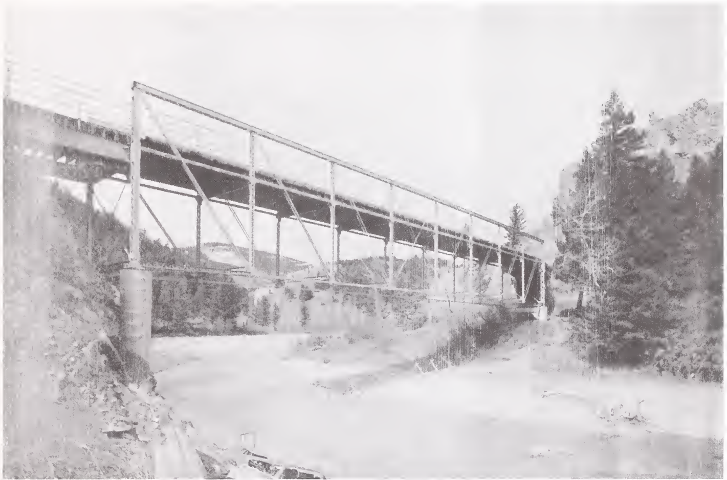
The Dearborn River High Bridge (HAER photograph by Jet Lowe).
